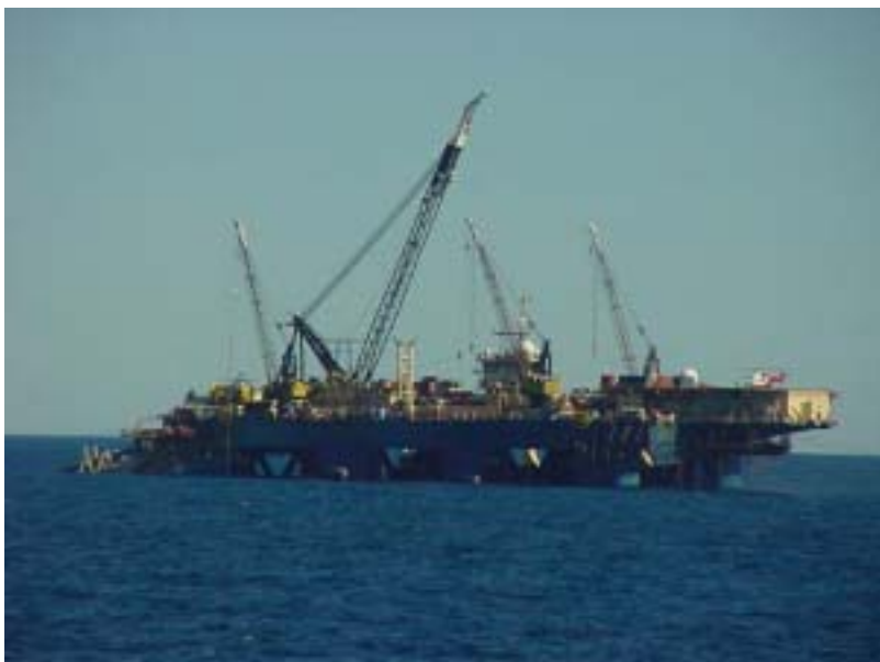
Semisubmersible pipe laying barge "Semac 1"
