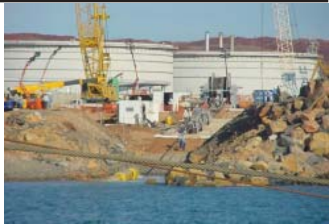
The pipe end going ashore in Withnell Bay
