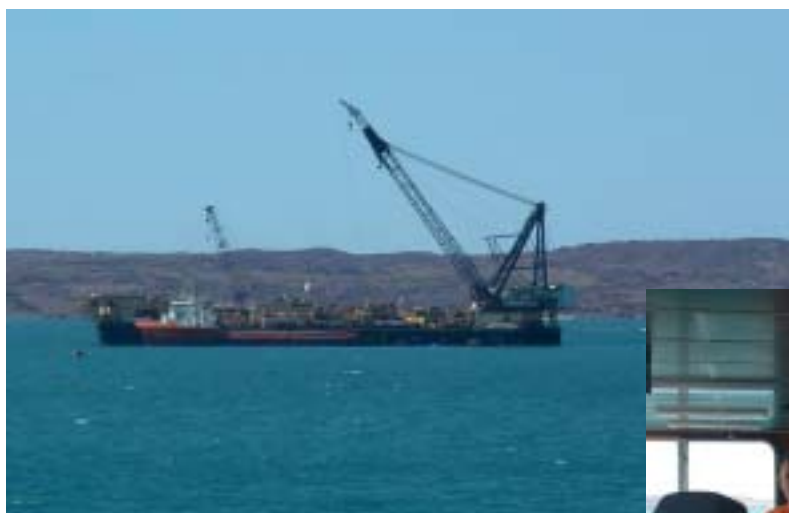
Above: Shallow water lay barge “Castoro 2” with “Pacific Spear ” alongside
